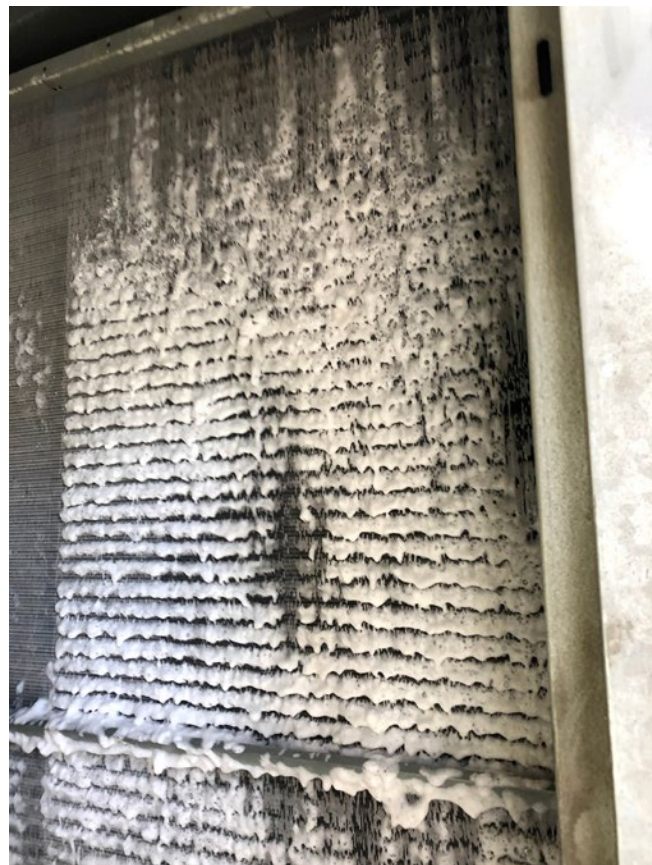
Biofilm buildup on HVAC coils can harbor and spread bacteria and viruses throughout the building.
