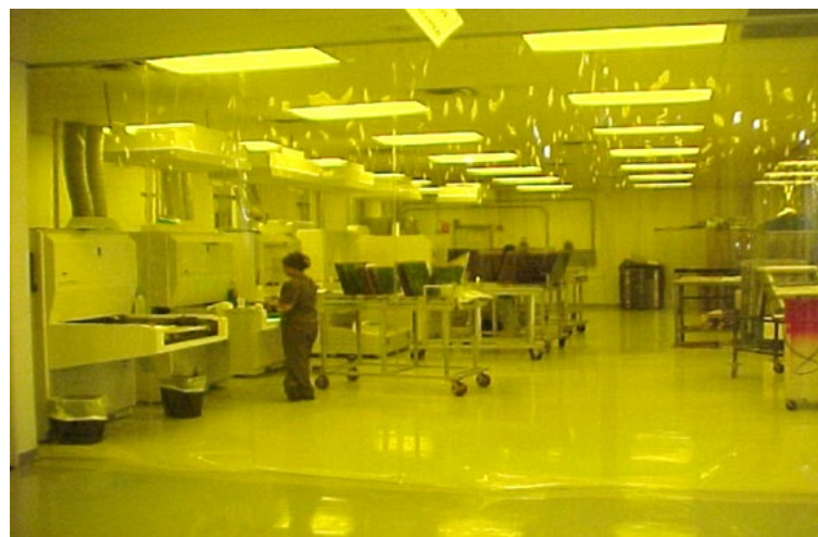
Figure 1: Cleanroom with curtains and HEPA filters in place (odd points of light are reflections).
