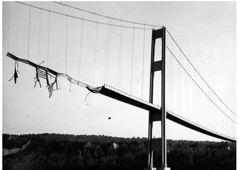
Tacoma Narrows Bridge during wind storm, known locally as "Galloping Gertie." Photo: Washington State Department of Transportation Special Collections Nov. 1940
